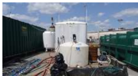
LNAPL SEAR Project: Injection of 260,000 gallons TASK™ ASB/polymer formulation, followed by 780,000 gallons of water, and recovery of same with LNAPL.
